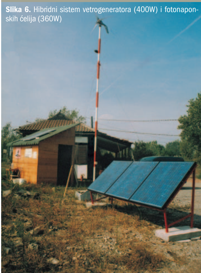
Figure 6. The hybrid system of the wind turbine (400W) and PV modules (360W)
